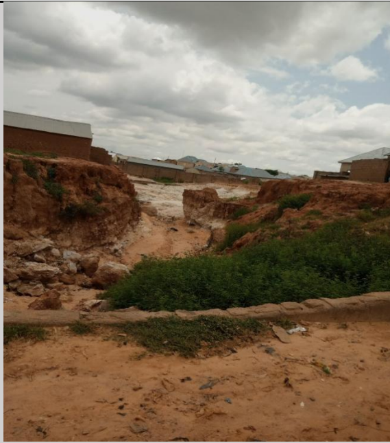
Figure 2.3: FCE (Technical) erosion site (Sub catchment 1 main gully upstream beginning at London Mai-dorowa)
